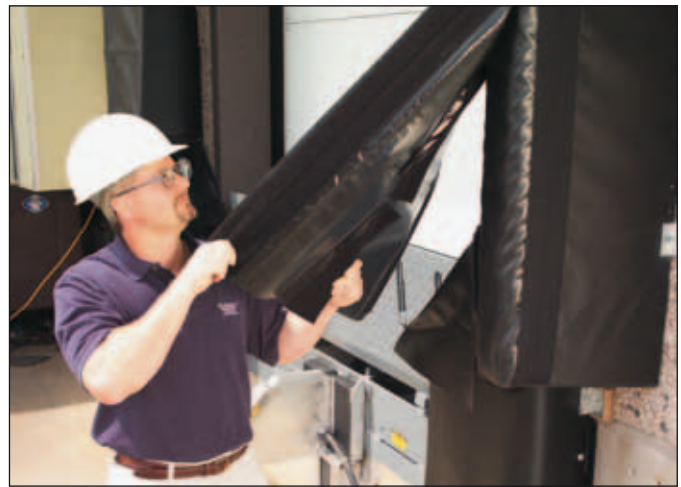
Gaps are sealed with Eliminator-GapMaster, without restricting access to the trailer
