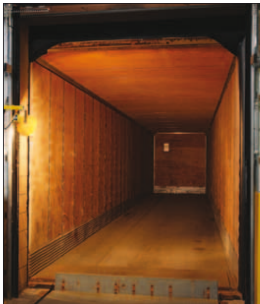
Incandescent 150 watt dock light
